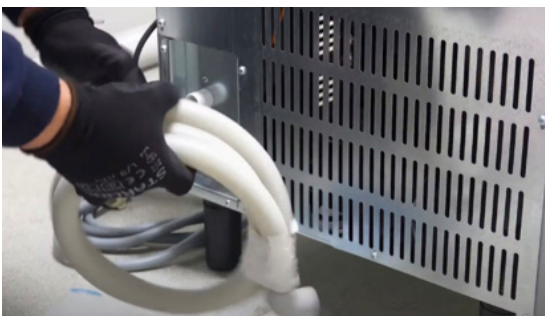
Fix water drain hose, assure it slopes downwards at least 15%
